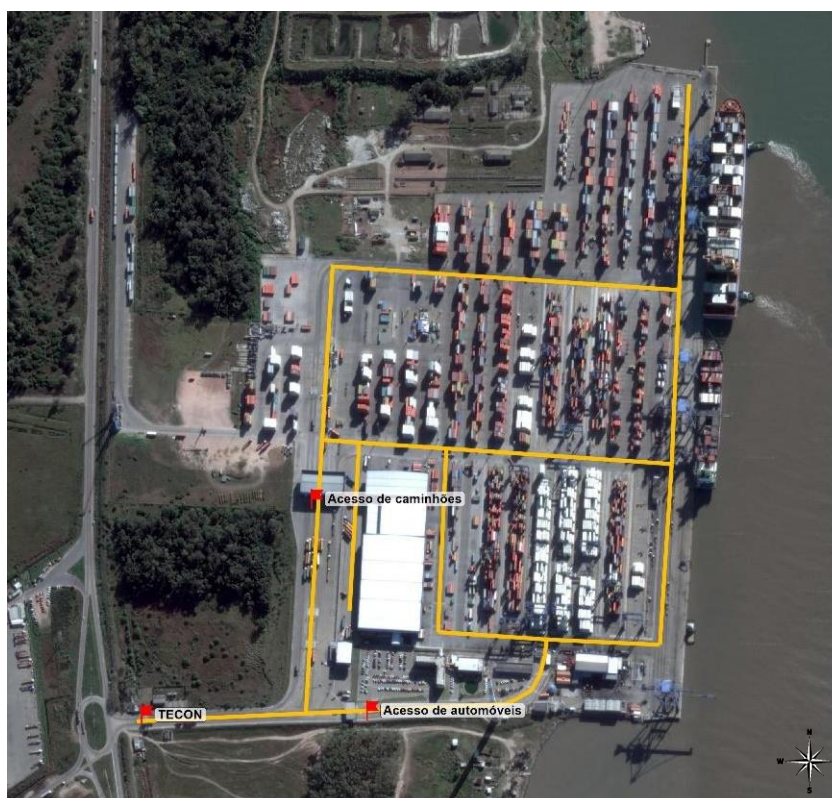
FIGURA 30 – Gates do Terminal Tecon
